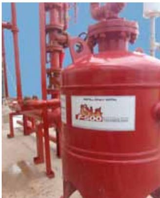
HCT engineers and packages Concentrate Control Supply (CCS) systems to precisely proportion F-500 Encapsulator Agent into the fire suppression system water stream. These systems typically include a bladder tank or other water-driven proportioning system, sized to maximize sprinkler and spray mist system effectiveness.
