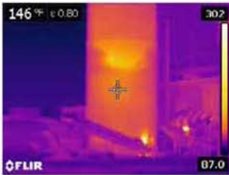
Cement silo fire, internal temperatures double readings on camera.
