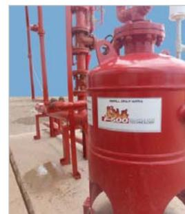
surfaces but is not effective on three-dimensional fires, like turbines. In fact, NFPA 11, Annex A.1.1. states, "Foam is not suitable for three-dimensional flowing liquid fuel fires or for gas fires."
