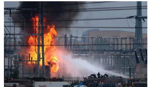
After receiving word from ConEdison, firefighters began applying Purple K to the transformer from two lines, but it kept re-igniting. So they applied foam and Purple K, but it continued to re-ignite. After 1 1/2 hours, they tried F-500 Encapsulator Agent, mixed with water at 3% through a single hand line. Since F-500 EA has the ability to cool the massive metal transformer and encapsulate the oil, F-500 EA extinguished the fire in less than two minutes.
