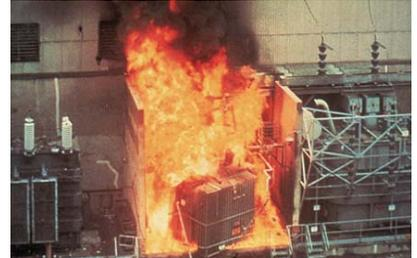
NFPA 11, Annex A.1.1 states, "Foam is not suitable for three-dimensional flowing liquid fuel fires or for gas fires."
