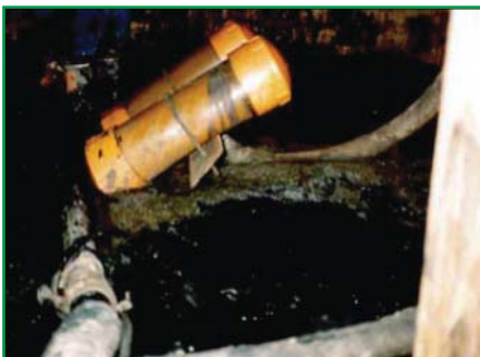
Before HydroLock Degassing and Cleaning
