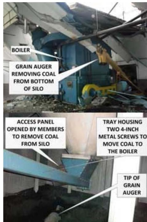
**Photo 5. Grain auger used to remove coal before explosion.
