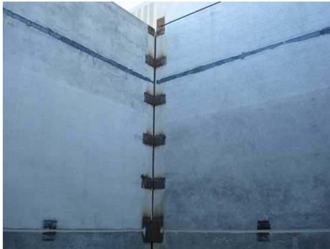
**Photo 1. Weld points to hold the panels together in a similar silo. The black metal strip going around the top two sections in the picture is the 4-inch weld strip for the sheet metal funnel transition panels for the corners.**
