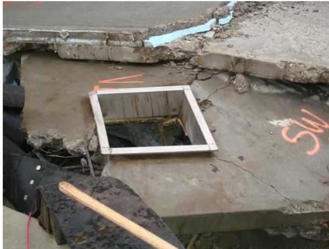
**Photo 4. Shows access panel on top of silo where the victims were flowing water at time of explosion.
