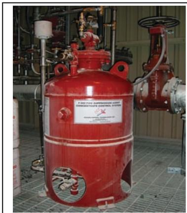
HCT engineers and packages Concentrate Control Systems to precisely proportion their F-500 Encapsulator Agent into the fire suppression system water stream. These systems typically include a bladder tank or other water-powered proportioning system, sized to maximize sprinkler and spray mist system effectiveness.
